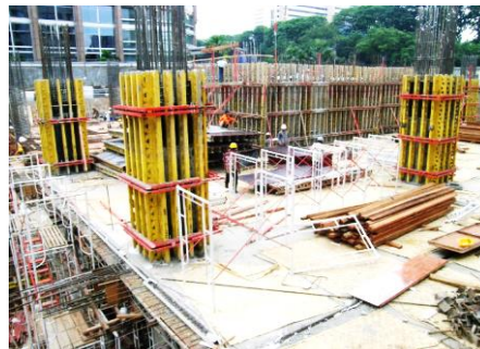
Gambar 7. Bekisting konvensional (Sumber : strong Indonesia.com)
